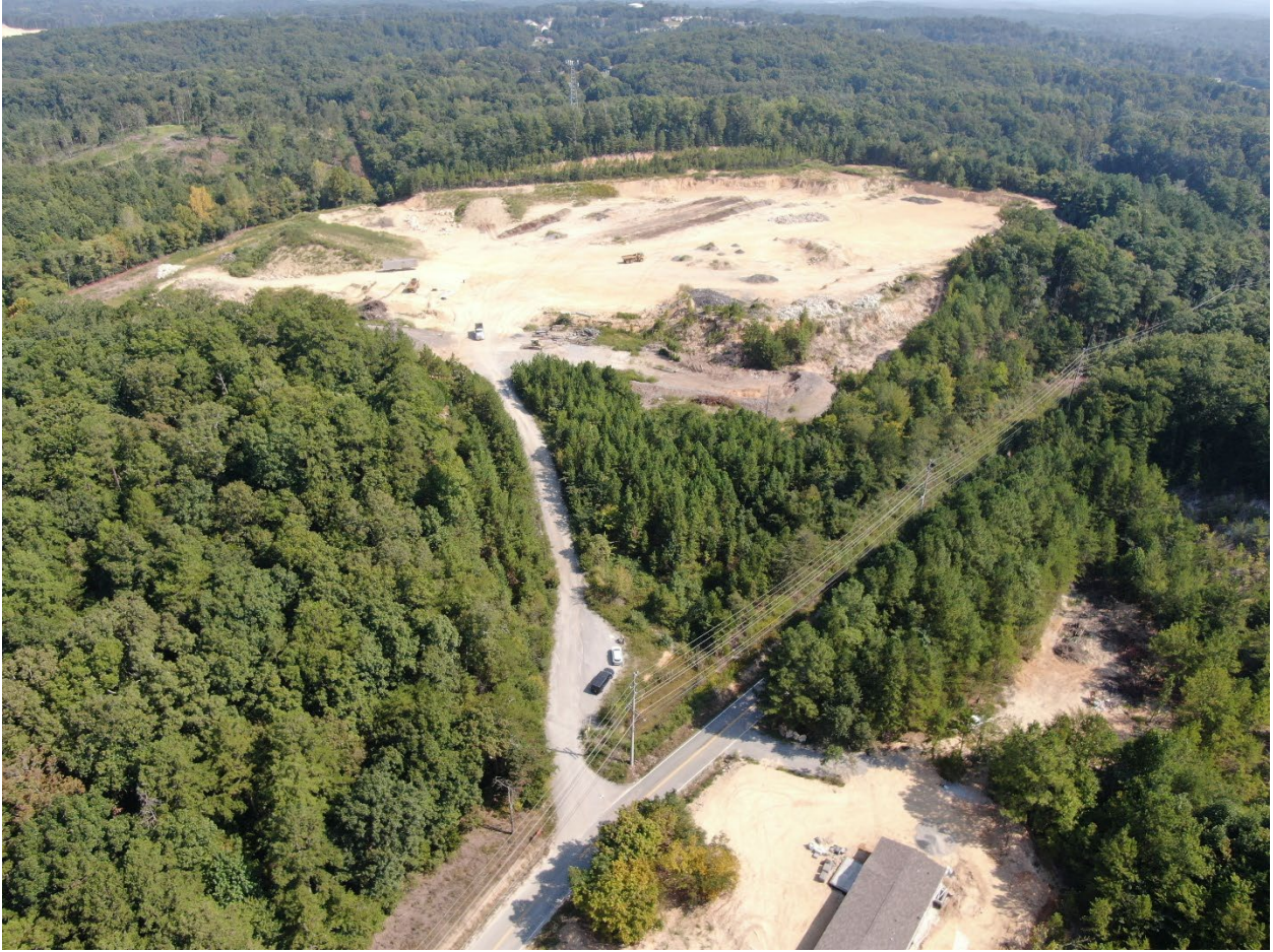
DRONE VIEW OF SITE
