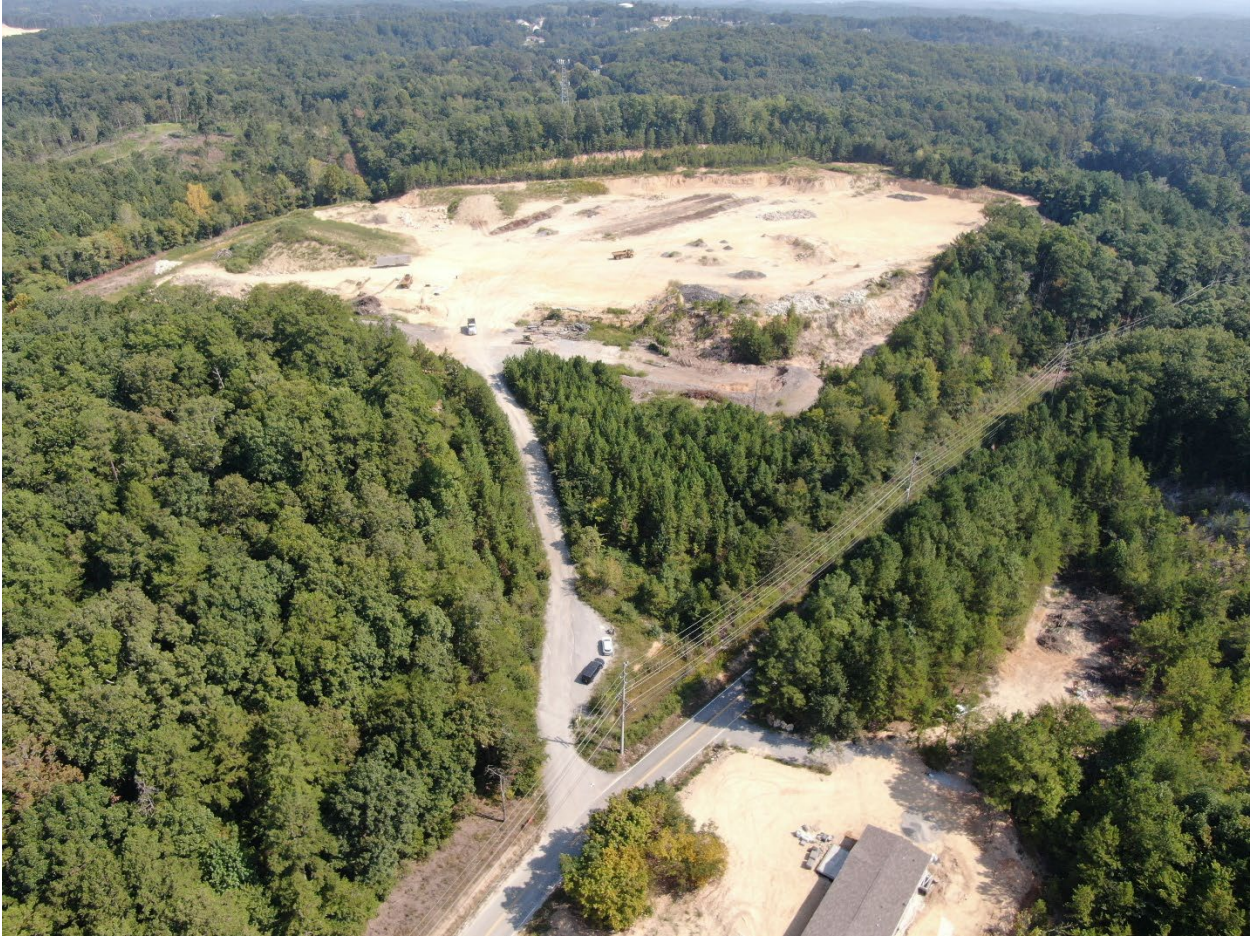
DRONE VIEW OF SITE
